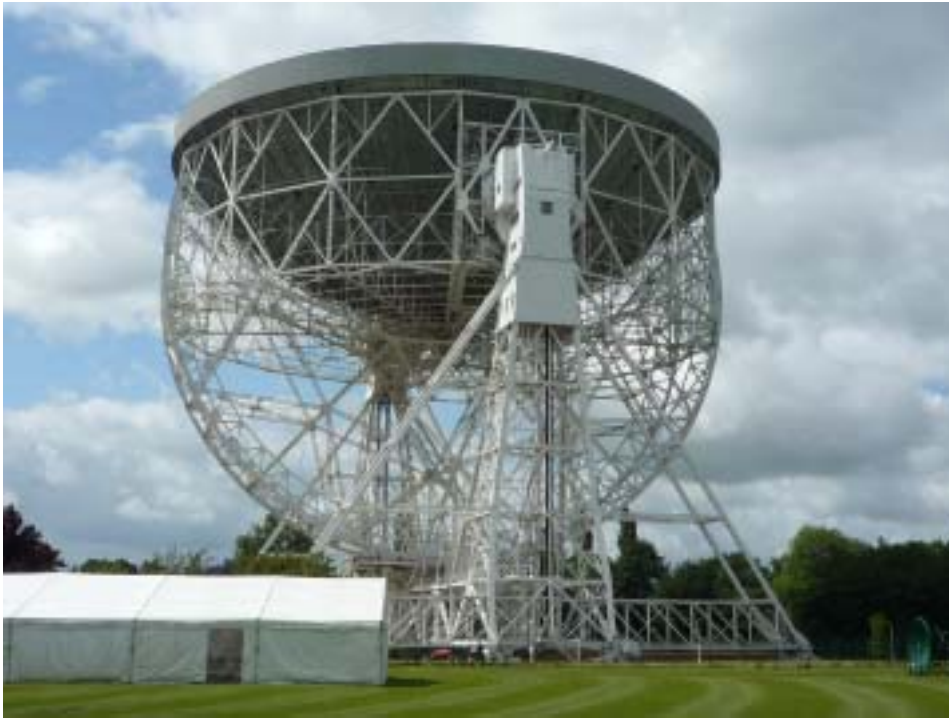
The main antenna was in stow position, as it was being repainted. The broad rim is part of the new, higher-gain dish surface, which was added in 1967 as part of the Mk. IA upgrade.
