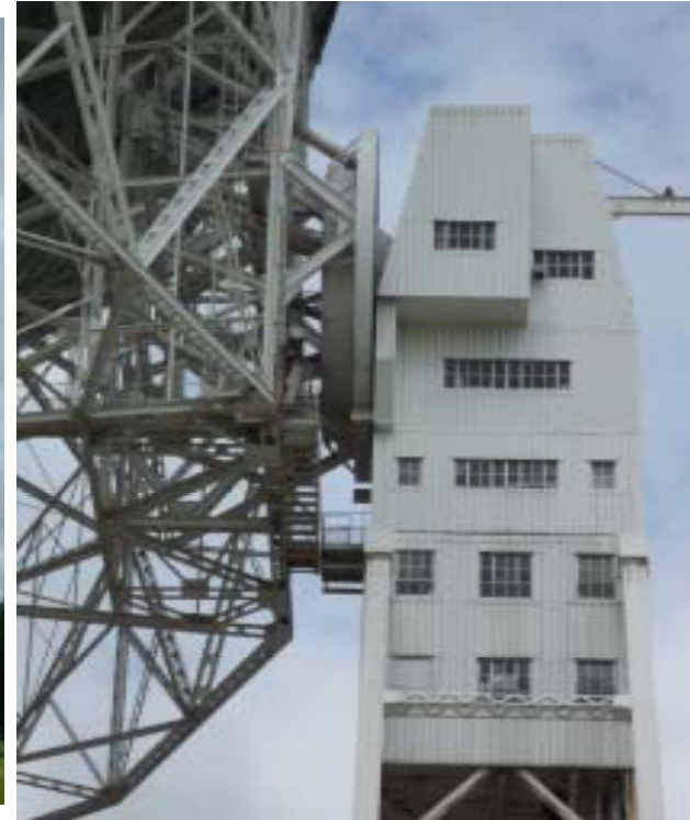
Detail of support tower housing elevation drive. The drives were taken from gun-turrets of scrapped Royal Navy warships.
