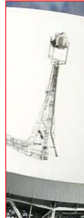
Detail of focus box and pylon. Note coax feedlines.
