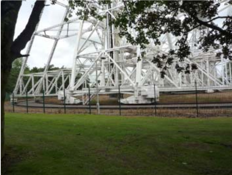
Detail of azimuth drive and track. The track diameter is 107.5m.
